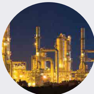
Energy and Industrial
